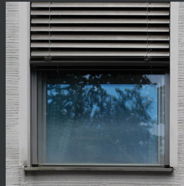
ELECTRIC EXTERNAL SHADING SYSTEMS
